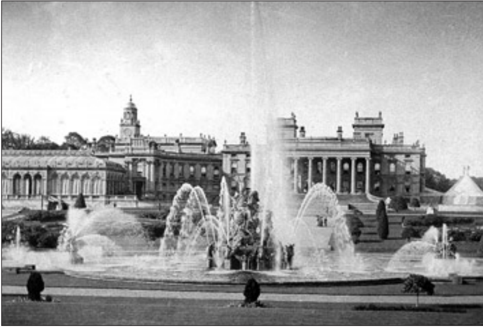
The Poseidon Fountain working in 1870. An immense amount of water was piped and pumped from pools and reservoirs as the main jet, which spouted from the sea monster's open mouth, reached a height of 36m (120ft). When the Dudleys were in residence, the fountains worked twice a week.
