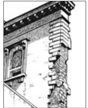
Jacobean red brickwork with Victorian Bath stone cladding
